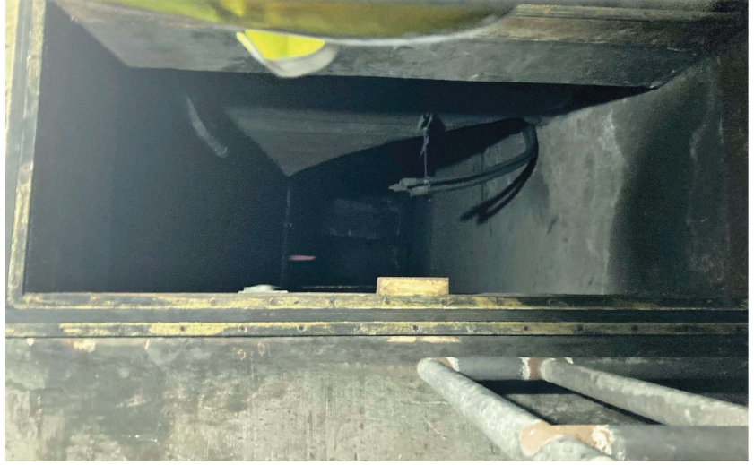
View of through plenum door into plenum.
